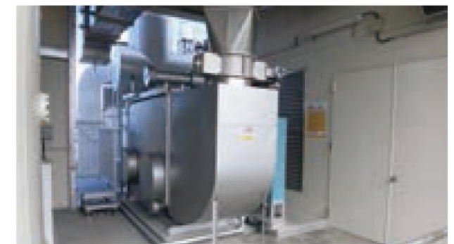
Gumma Works: Exhaust heat recovery boiler
