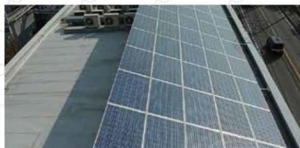
Solar battery panels installed on the roof of Yao Works
