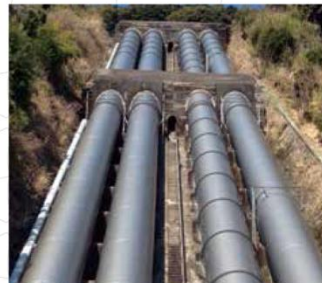
Penstock at Kambara Complex, Nippon Light Metal Company
