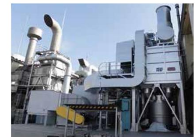
VOC treatment system at the Gunma Works
