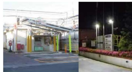
Carport equipped with Hane™ modules (left) and LED street lights (right) powered by the modules at the Yao Works
