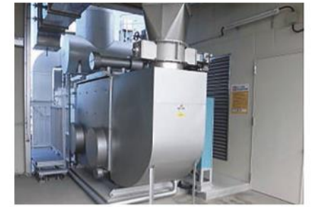
Exhaust heat recovery boiler in Gunma Works
