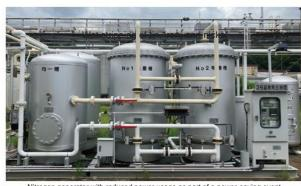
Nitrogen generator with reduced power usage as part of a power-saving e
