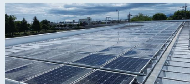
HaneModule, lightweight solar cell modules that weigh two thirds of conventional modules
