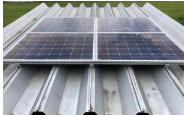
Fig. 1 Installation of the module onto corrugated roof
