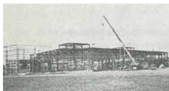
Gumma Plant under construction
