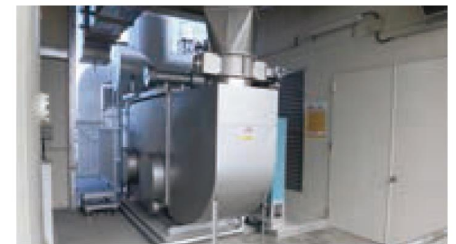
Gumma Works: Exhaust heat recovery boiler
